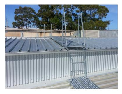
Our Galvanised walkways have non-slip, raised 40mm x 12mm surface openings grip the sole of any work boot / shoe in all directions, minimising the risk of slipping even in the harshest of conditions.
